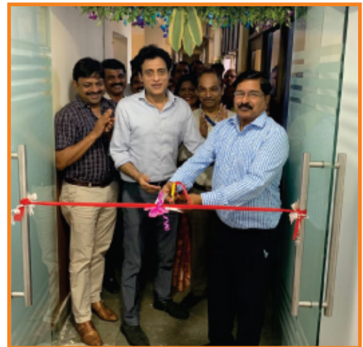
Unveiling of new container terminal data centre at JNPT
