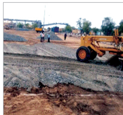
Paved Storage Yard – work in progress
