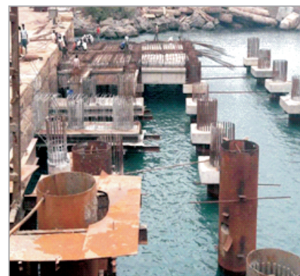
Piling work in progress
