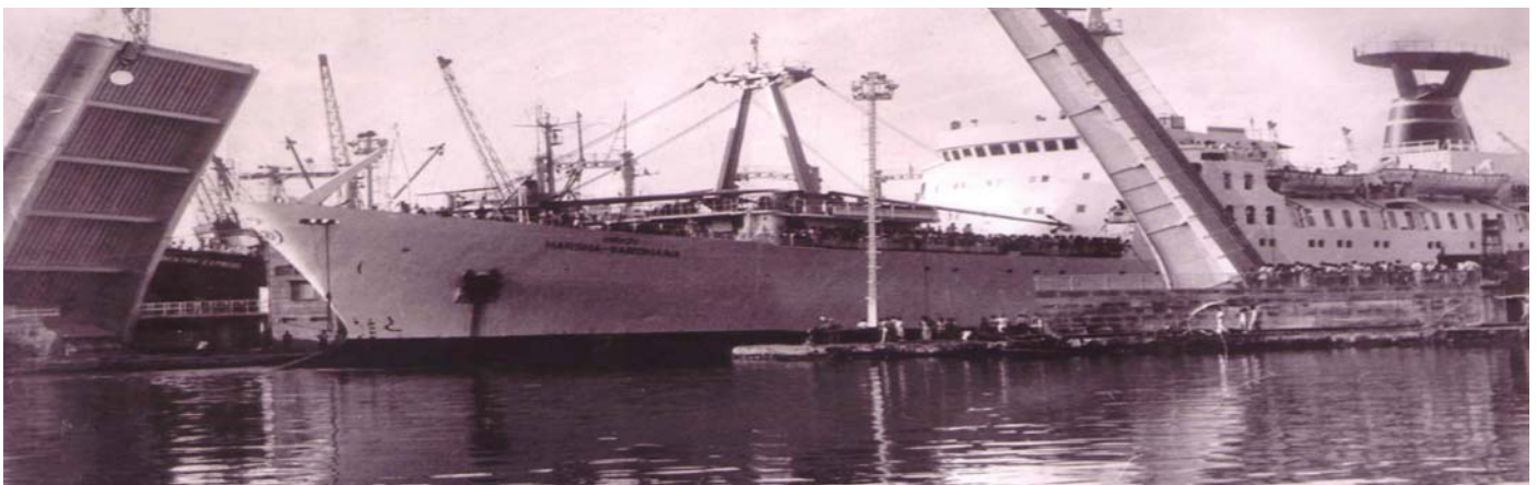
The swing bascule bridge at Kidderpore
