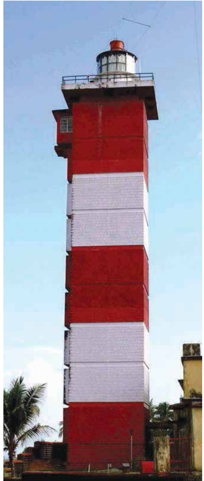
Suratkal Lighthouse: It is located north of port of Mangalore and is made of 36-meter-high square masonry tower with a luminous range of 31 nautical miles. The lighthouse tower was constructed in 1972. Differential global positioning system (DGPS) was established at this station in year 1998.
