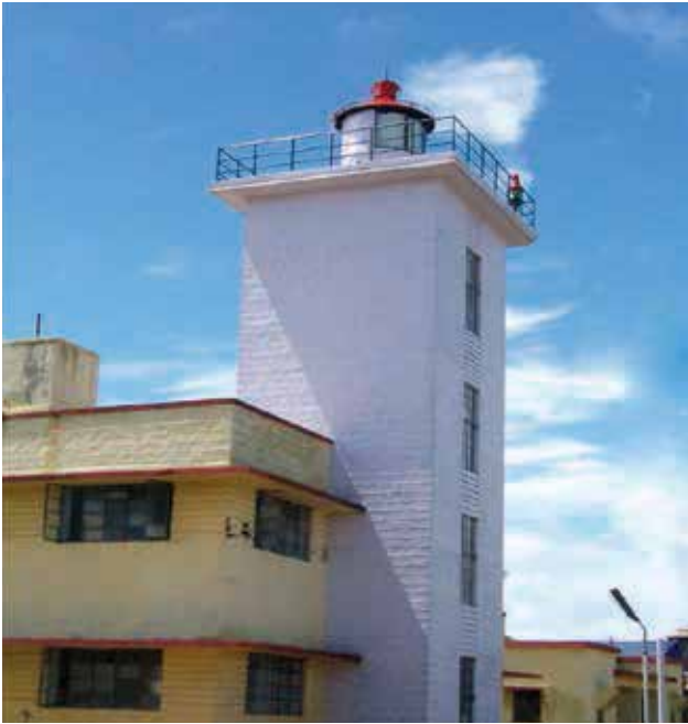
Bhatkal Lighthouse: Tucked away in a small town called Bhatkal, it constitutes a 14-meter-high, square masonry tower with a luminous range of 27 nautical miles. This stone masonry lighthouse was built in 1891 and subsequently modernized in 1995.
