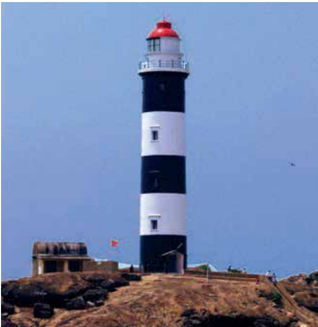
Kaup Lighthouse: A stunning architecture from another era, the lighthouse is in Muloor, about 12 km away from Udupi city, and is made of 34-meter-high circular stone masonry tower with luminous range of 24 nautical miles. It was built by the British in 1901 and subsequently modernized in 2003-04.
