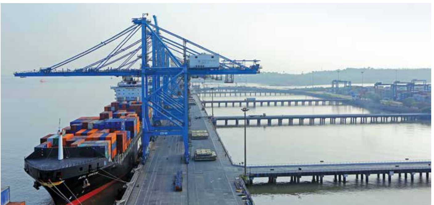
Docking of a container ship at JN Port
