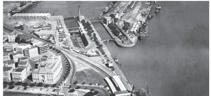
Aerial view of the Alexandra Dock and the Hughes Dry Dock
