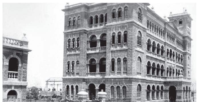
Old Port House. Vijaydeep Annexe Building was constructed in 1965
