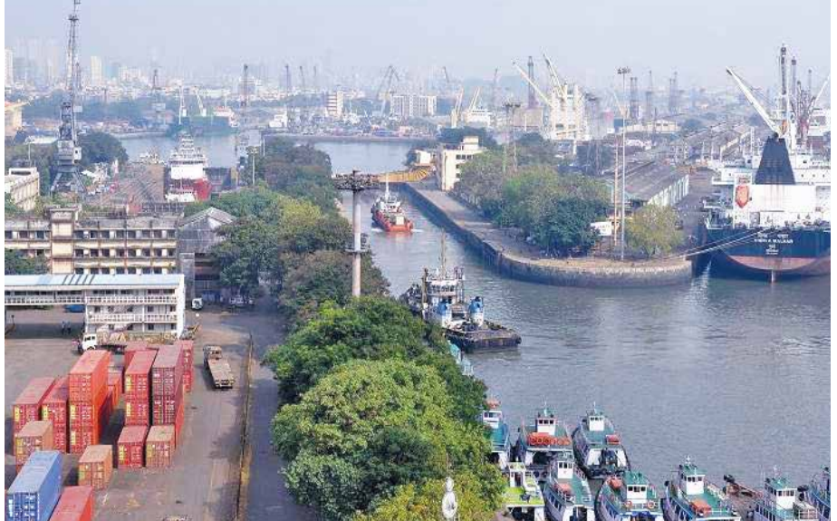
An aerial view of Mumbai Port
