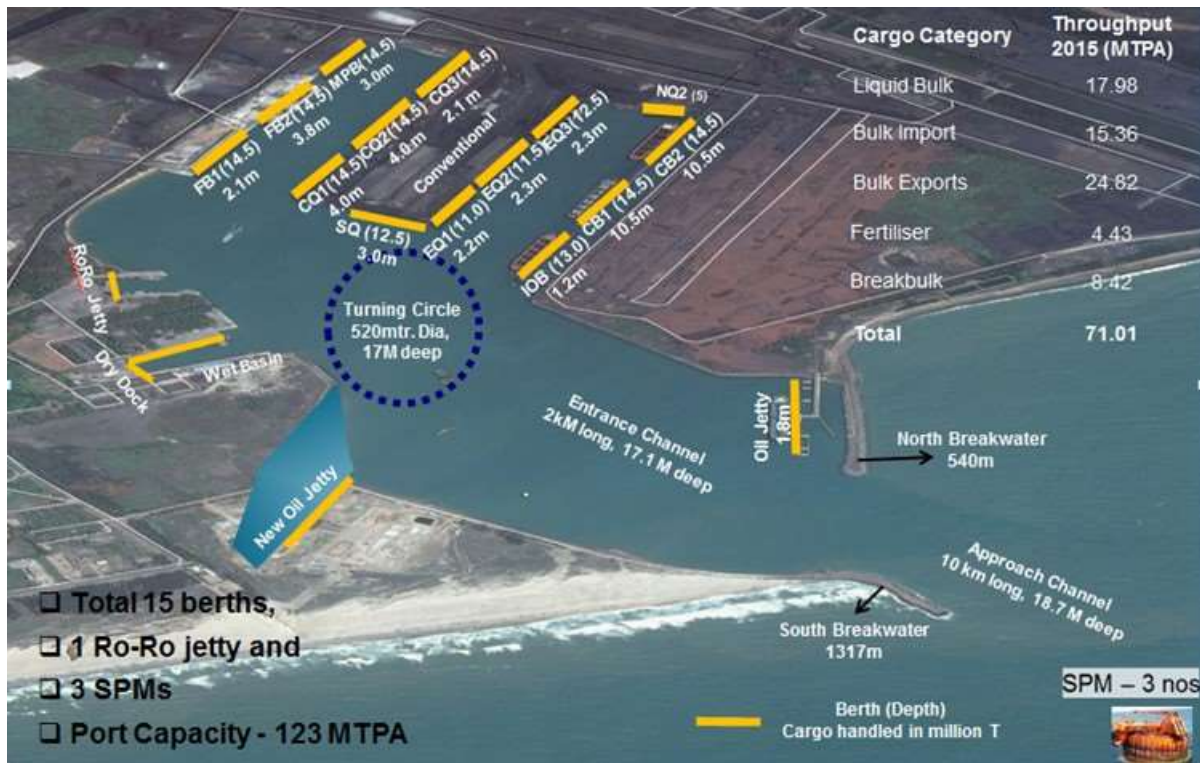
Figure 2.2 Existing Facilities at Paradip Port
