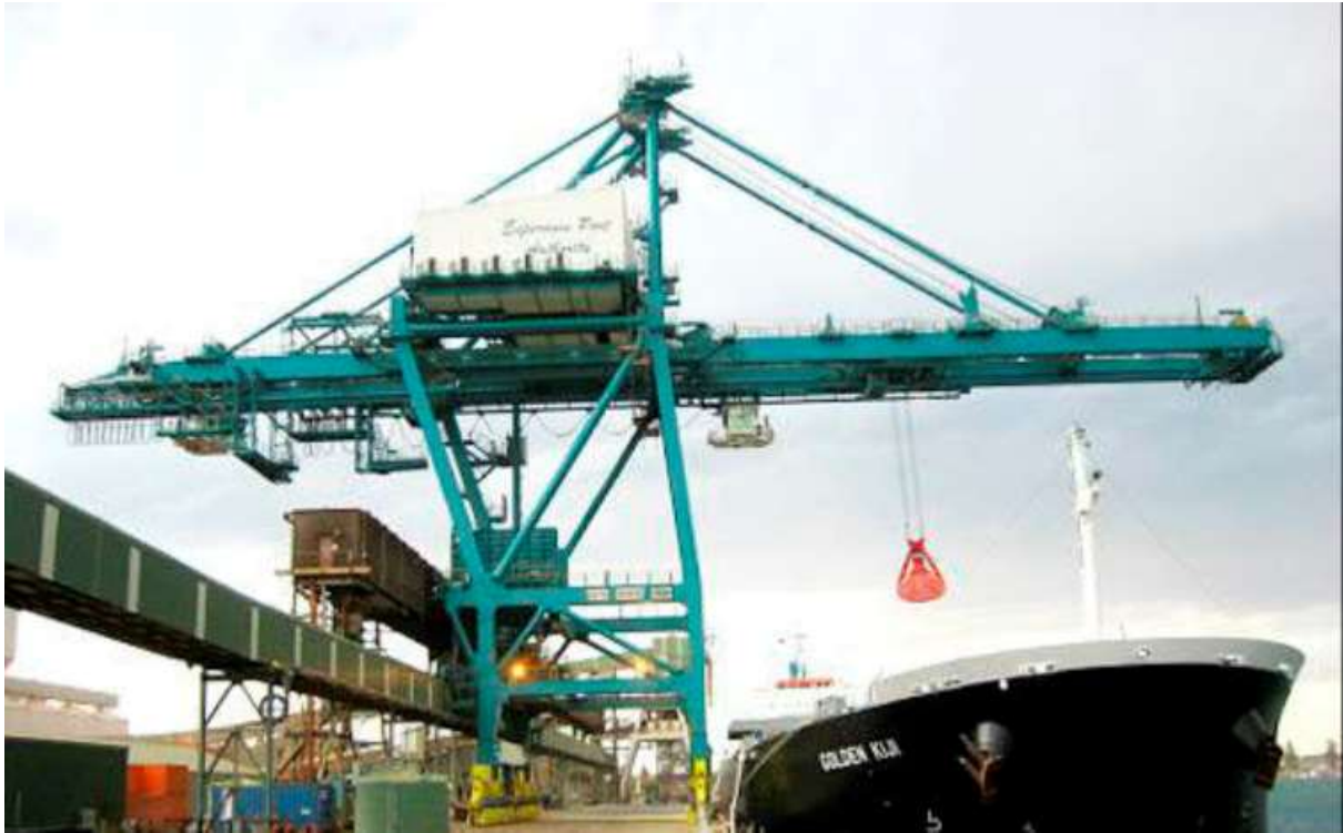
Figure 8.14 Typical Gantry Type Ship Unloader
