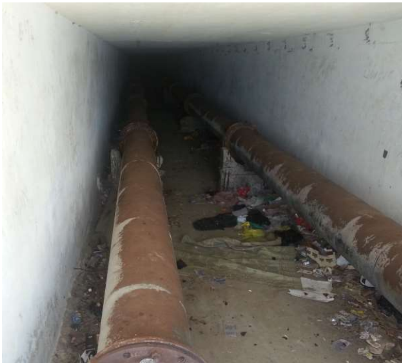
Figure 4.3 Submarine Tunnel with 2 x 15" Pipelines
