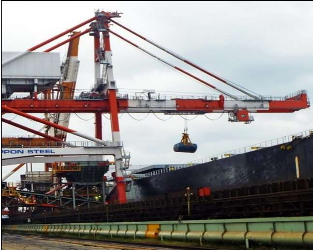
Figure 7.23 Typical Ship Unloader
