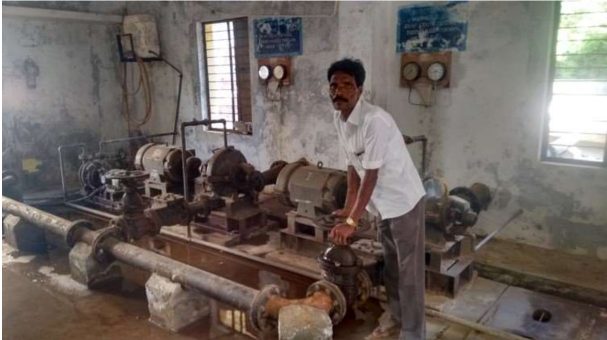
Figure 3.12 Existing Water Supply Station
