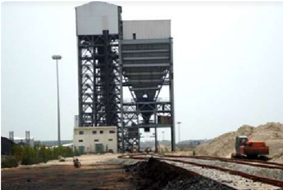
Figure 8.16 Typical Rapid Loading System
