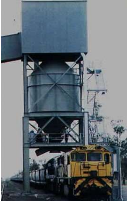
Figure 7.25 Typical in-motion Wagon Loading System
