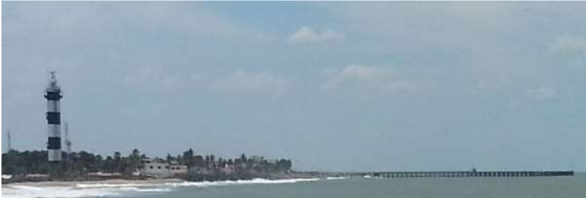
Figure 2.4 View of the Piled Jetty & Light House
