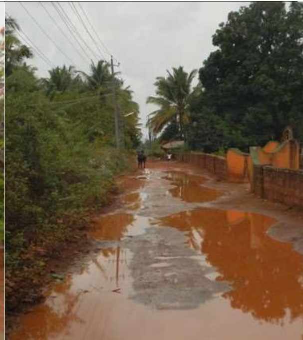
A. Road to Keni village (Project site); kutcha road (3-4 m); agriculture land on both sides
