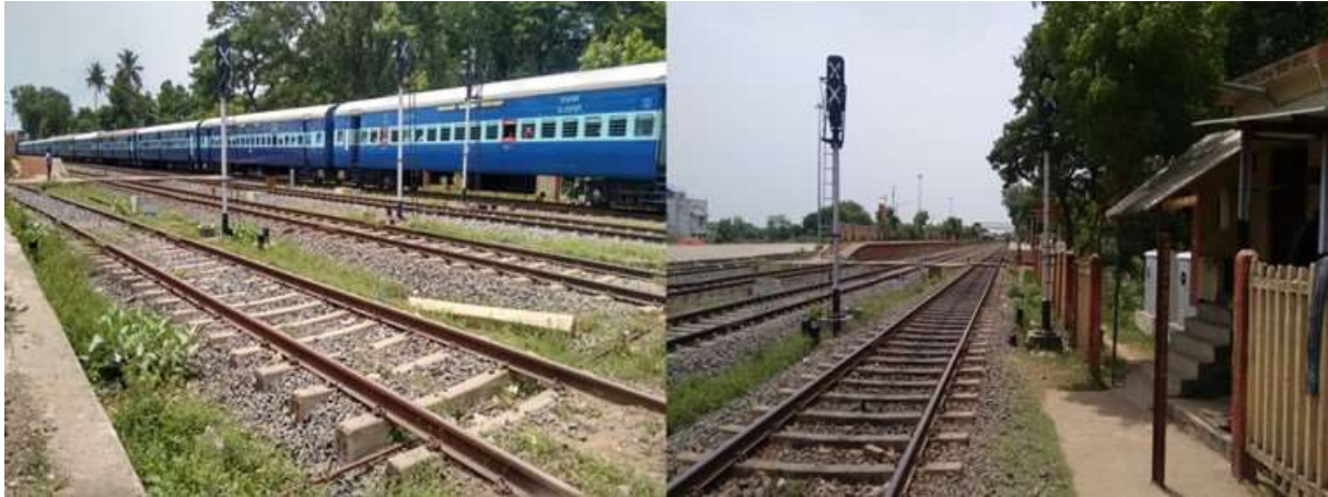
Figure 3.8 Sirkazhi Railway Station at Present
