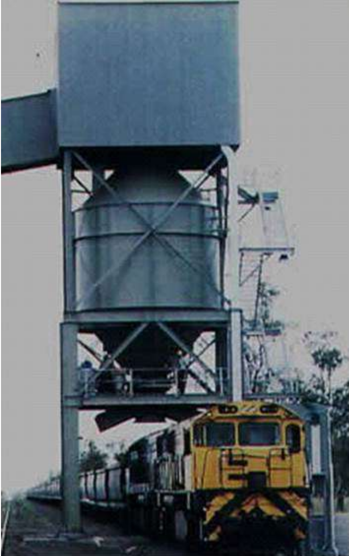
Figure 7.3 Typical in-motion Wagon Loading System
