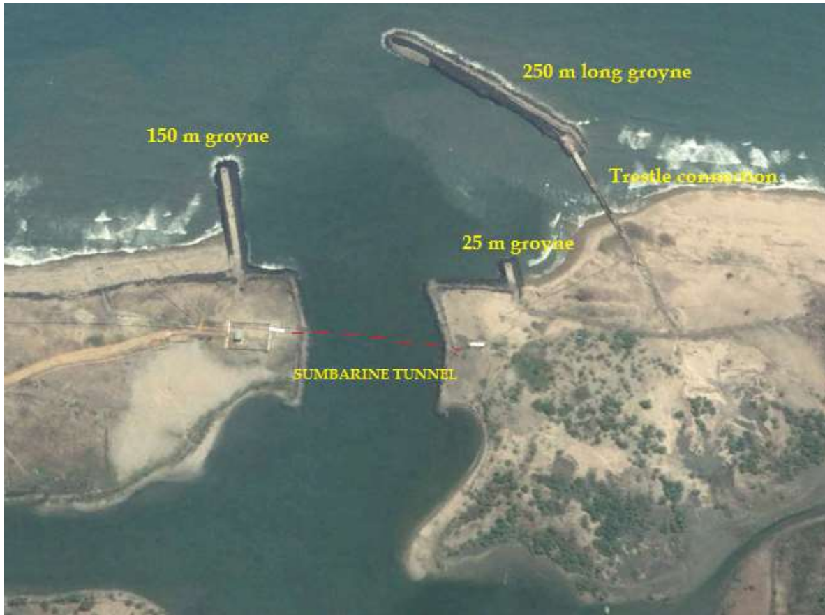
Figure 2.5 Structures at the River Mouth
