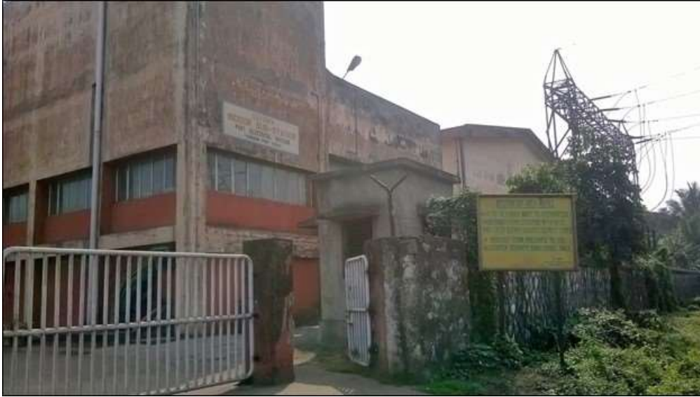
Figure 2.21 Electrical Substation at Paradip
