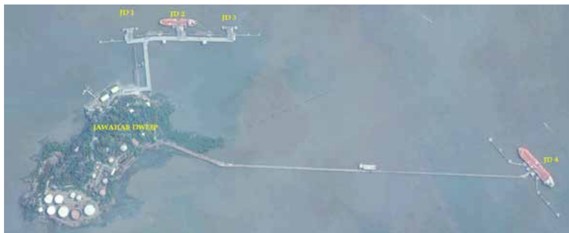
Figure 3.6 Marine Oil Terminal at Jawahar Dweep
