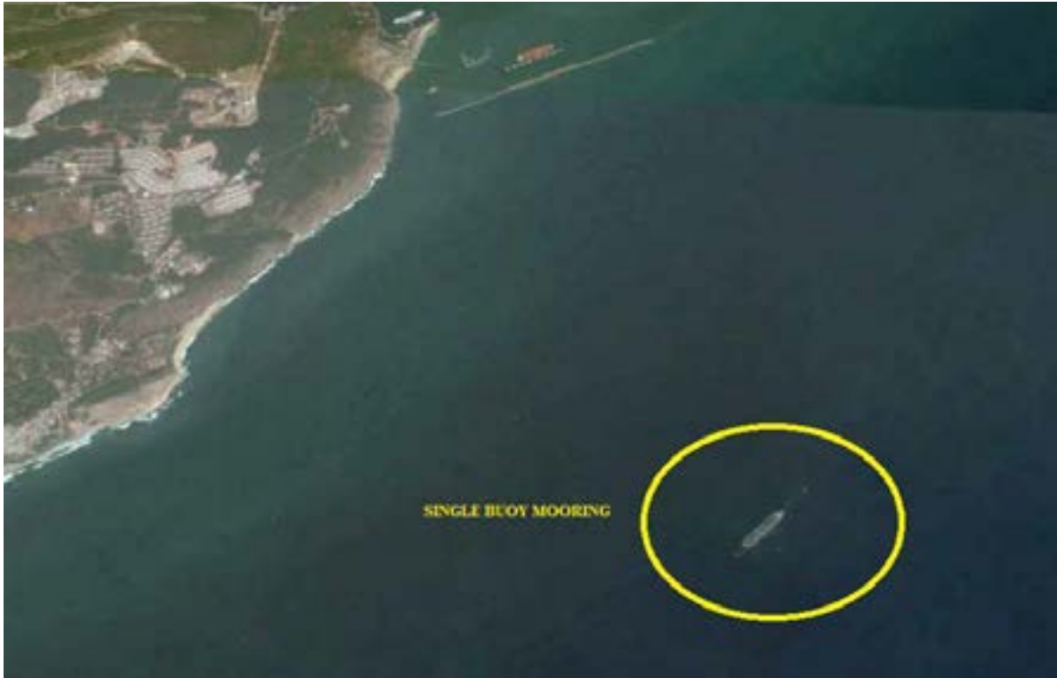
Figure 3.9 Relative Location of VPT Eastern Breakwater and the SBM
