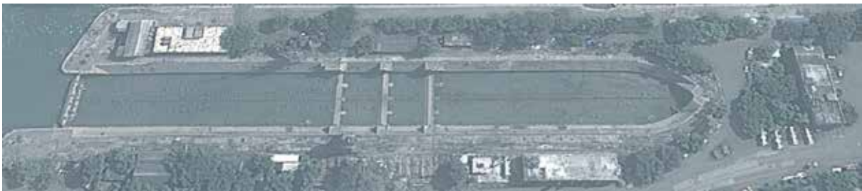
Figure 3.9 General View of Hughes Dry Dock
