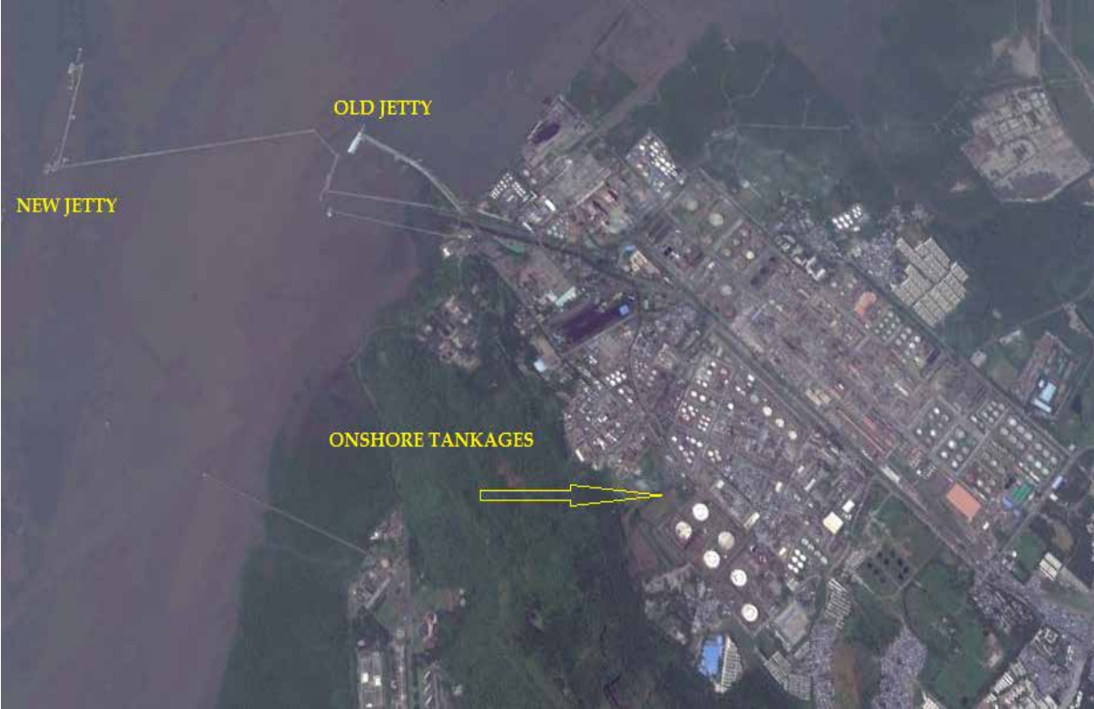
Figure 3.7 Chemical Terminal at Pir Pau
