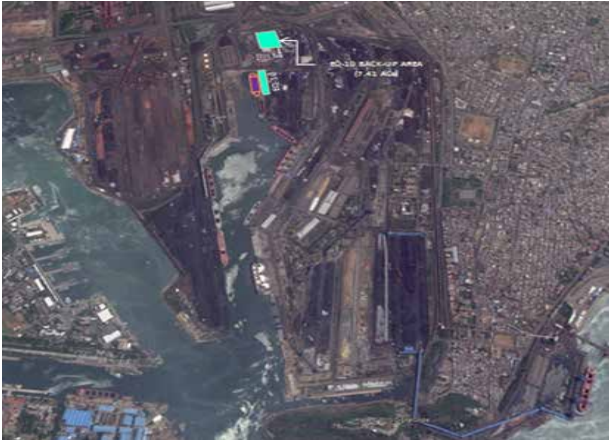
Figure 3.2 Berth with the Backup Area
