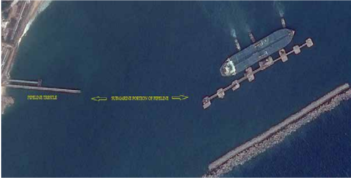
Figure 3.7 The Offshore Tanker Terminal and the Pipeline Trestle
