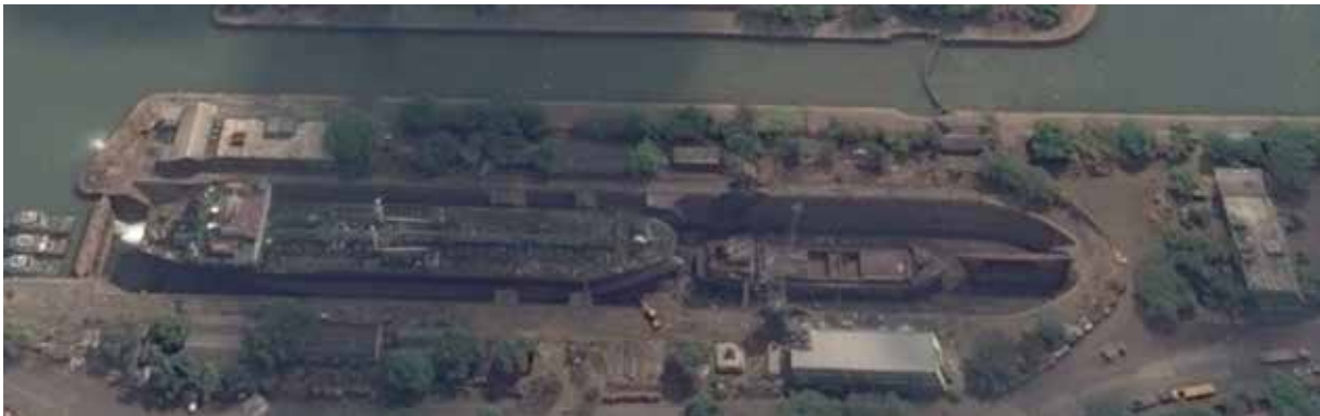
Figure 3.10 View of Dry Dock with Two Vessels Docked
