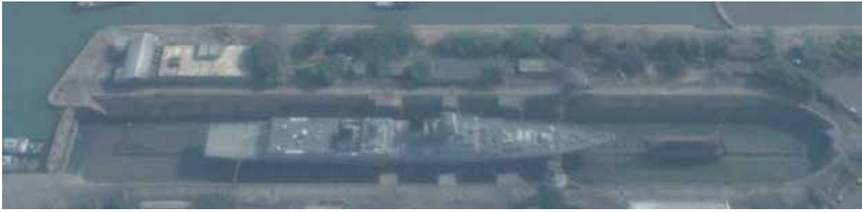
Figure 3.12 View of Dry Dock with Single Vessel Docked
