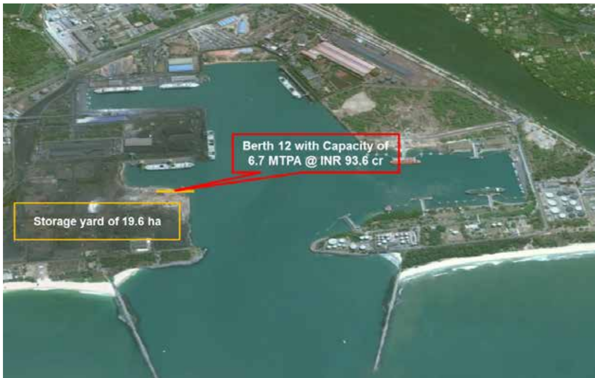
Figure 5.1 Mechanisation of Berth 12
