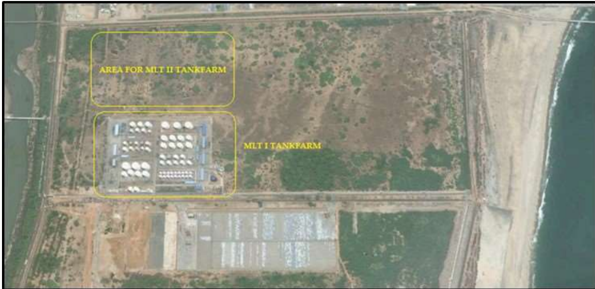
Figure 7.7 MLT 1 Tank Farm
