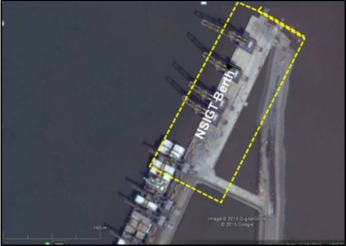
Figure 5.2 NSIGT-DPW's 330 m Container Berth, Approach Bund and Trestle
