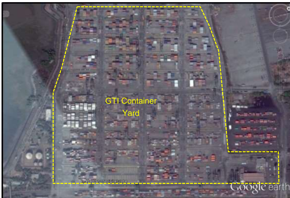
Figure 3.6 GTI Container Yard
