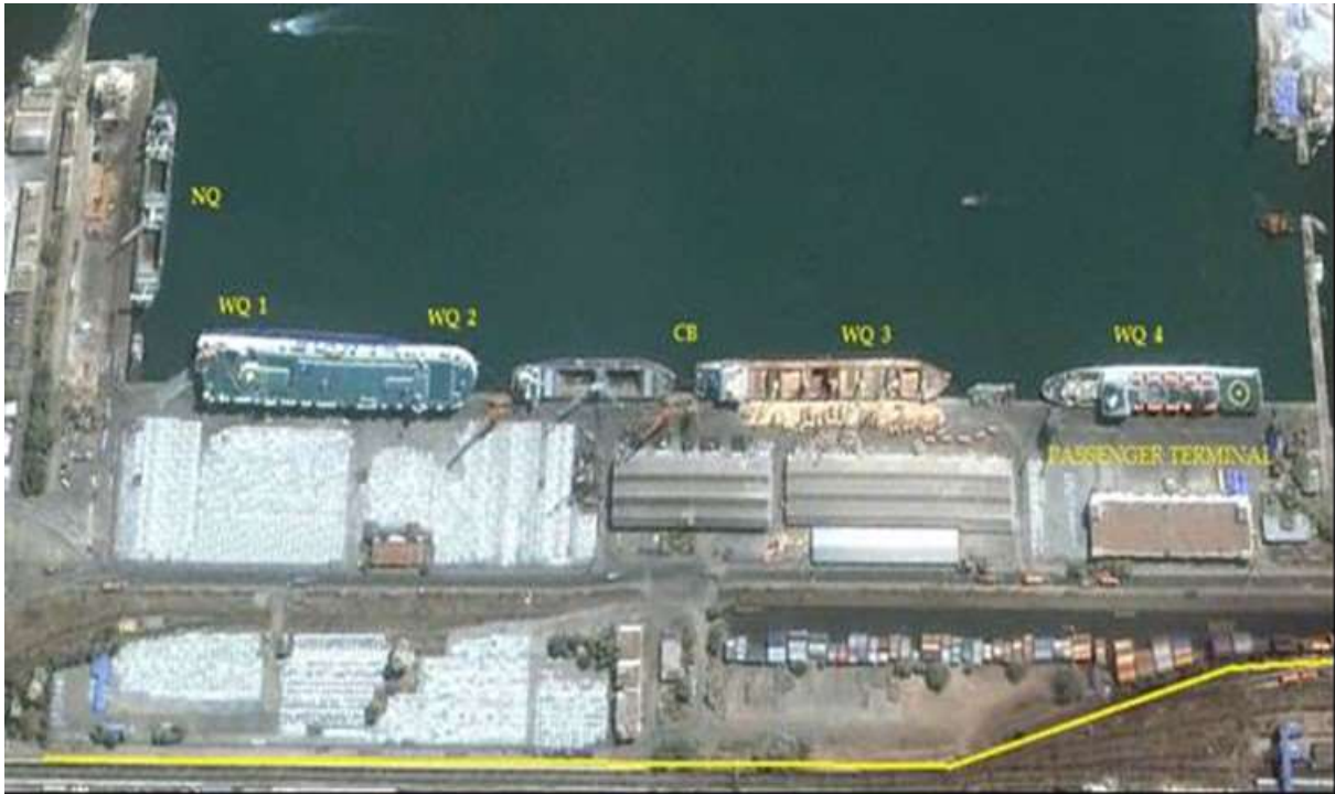
Figure 6.11 North Quay and West Quay Berths
