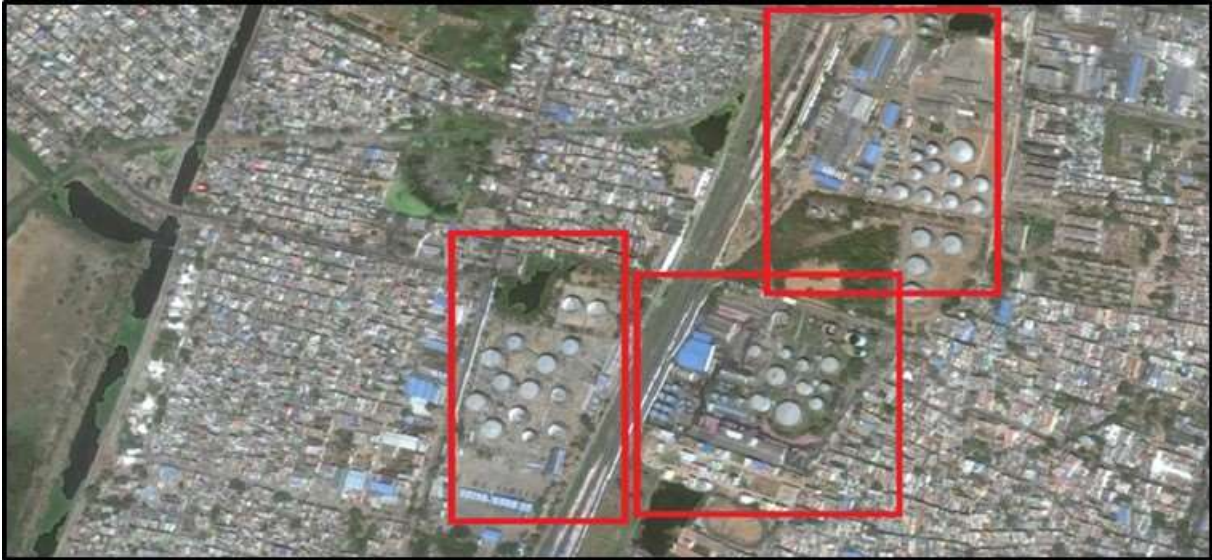
Figure 7.1 IOC, HPC & BPC Terminals in Crowded Tondiarpet – Korukkuppet Area of Chennai
