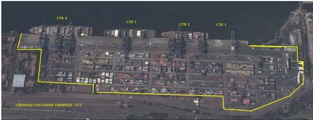
Figure 6.10 Chennai Container Terminal (CCTPL)
