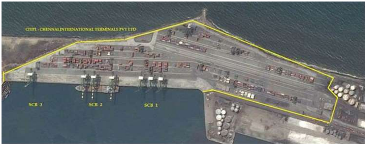
Figure 6.13 Chennai International Container Terminal (CITPL)
