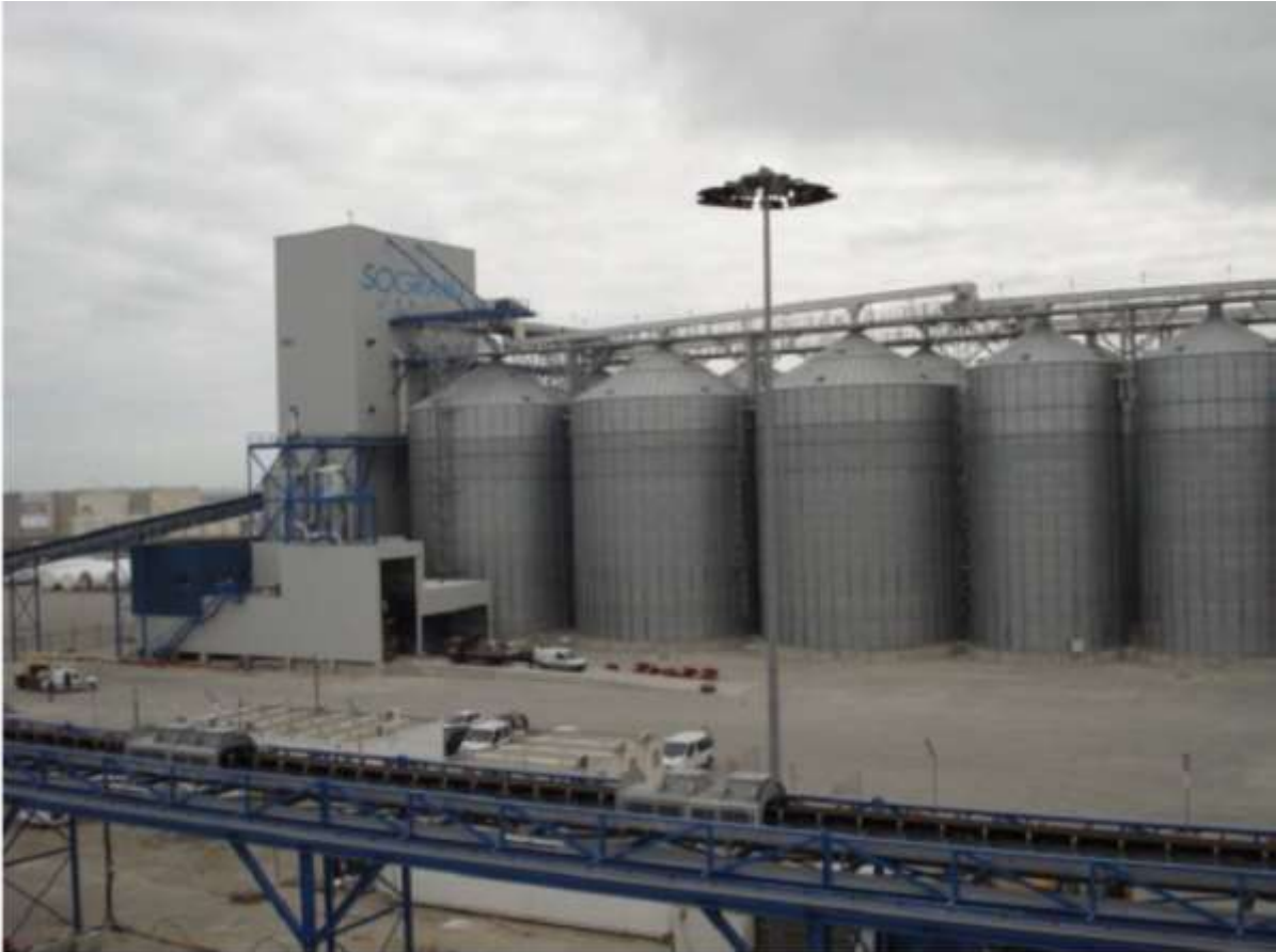
Figure 8.2 Steel Silos for Food Grains
