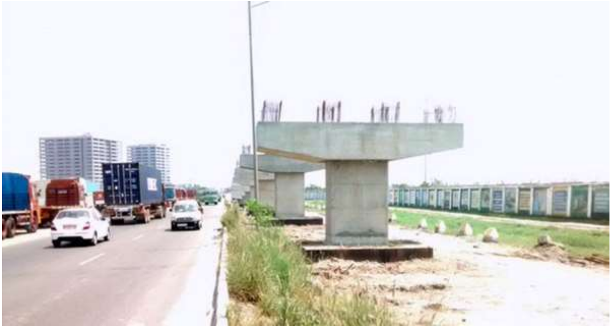
Figure 5.4 Construction of ROB to Ease Congestion
