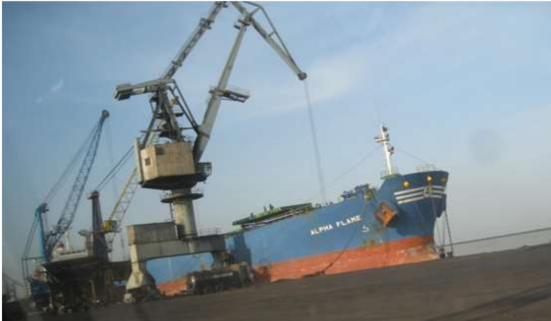
Figure 9.1 Coal unloading Facility through Multipurpose Berths
