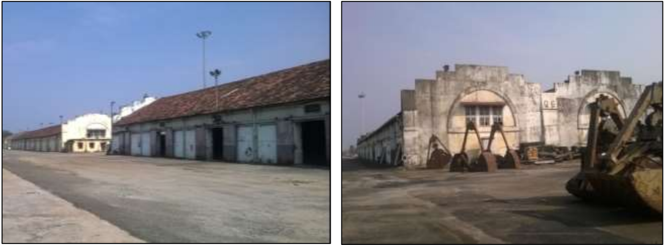
Figure 3.5 Storage Sheds at Mattanchery and Ernakulam Wharf
