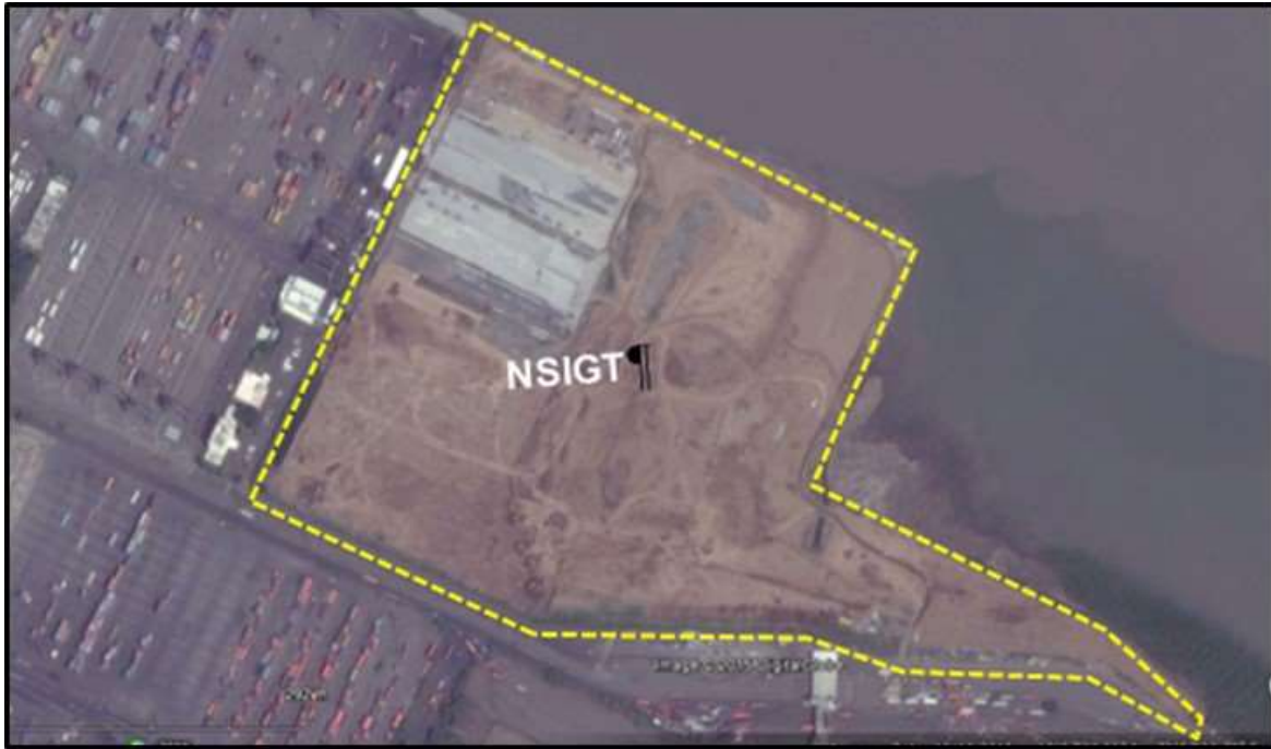
Figure 5.3 NSIGT-DPW's 330 m Berth Container Yard Under Development
