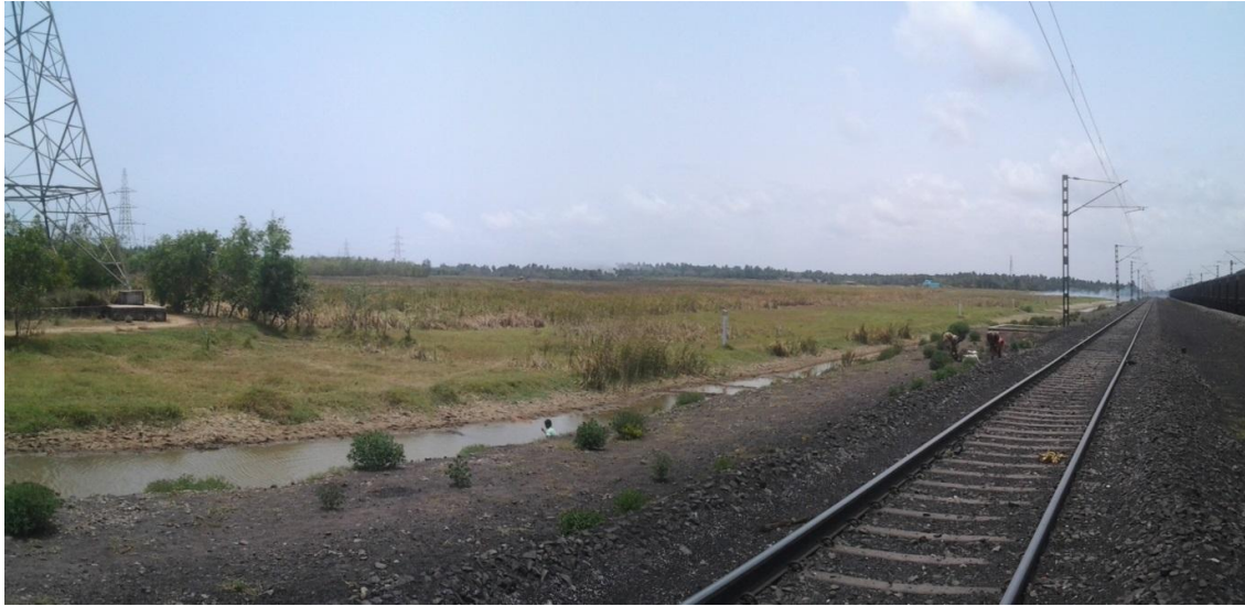
Figure 8.11 Land on the Other Side of DE for Haridaspur Track
